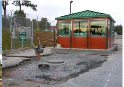
Septic Tank & Building
