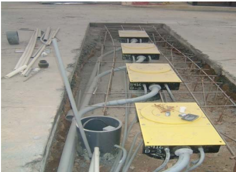
"Pop-Up" Bollards Installation
