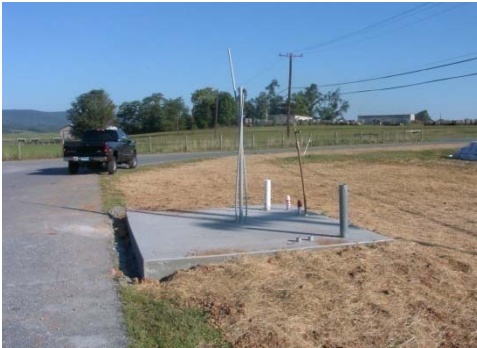
Concrete Pad & Utilities
