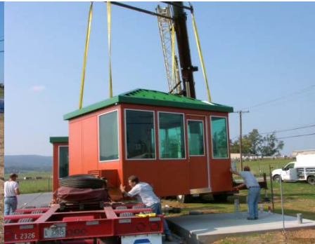
Unload & Set Building
