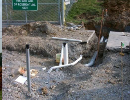
Plumbing Rough In
